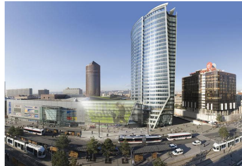
Figure 2 Part Dieu (France) commercial centre
